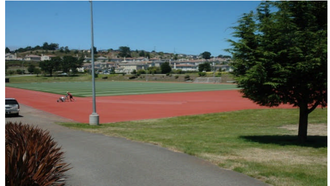
Skyline College Track Resurfacing
